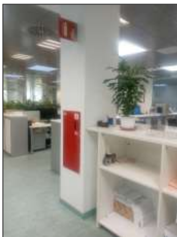
15 Extintor no visible
